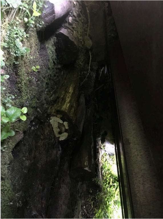
Left Bank Abutment when facing downstream
