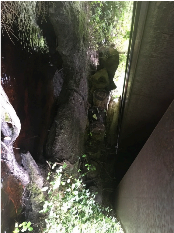
Right Bank Abutment when facing downstream
